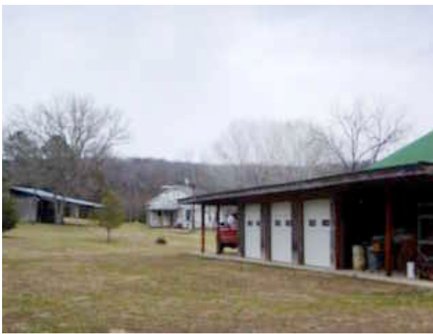
Looking from the power shed to the workshop and beyond to the house. Note the satellite dishes on the house.
