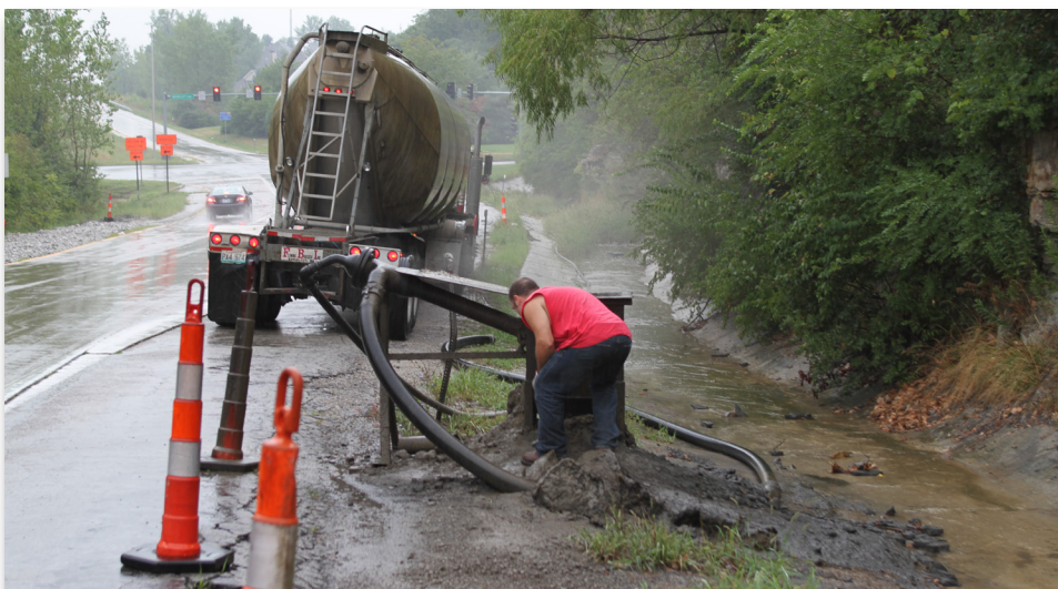
Coal ash being dumped in underground mines near Briar Cliff in Kansas City, MO Photo: Claus Wawrzinek
