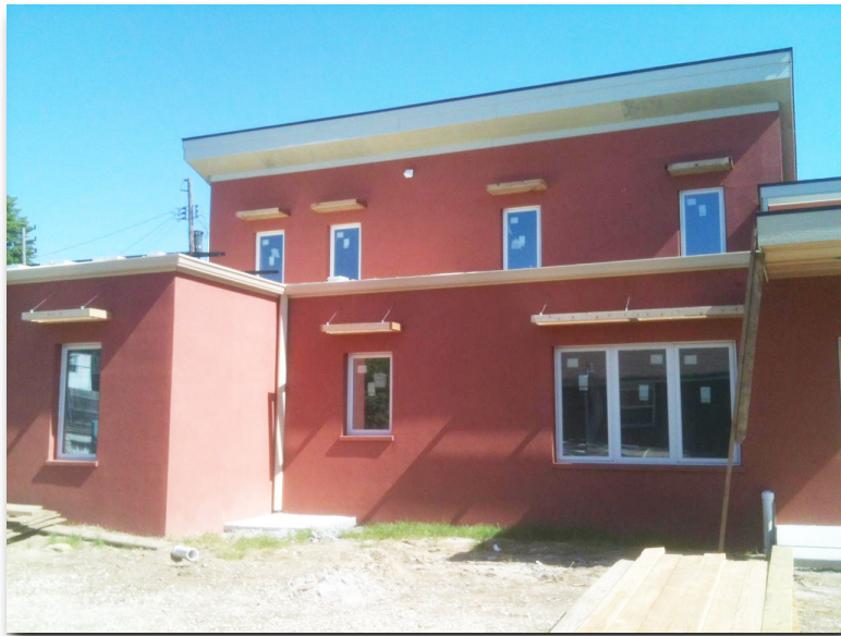
Dan and Michelle's new passive house under construction.
