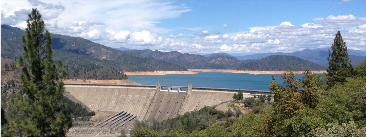
Federal officials say adding 18.5 feet to the top of Shasta Dam would enlarge the reservoir's capacity by about 14 percent. (Craig Miller/KQED)
