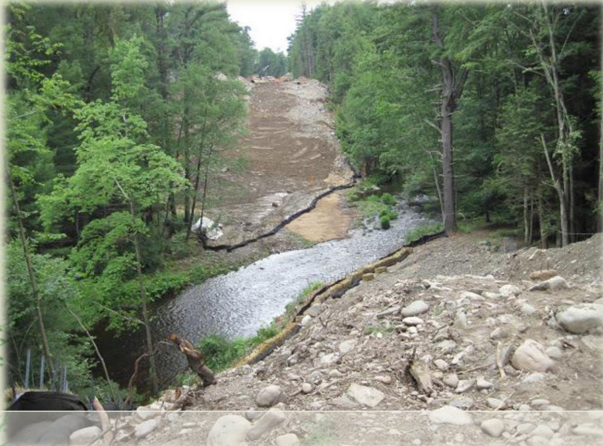
DRN, TGP Pike County, PA across the Sawkill Creek. June 2011
