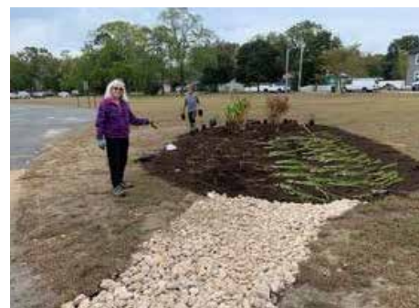
Volunteers plant the day after the basin is completed
