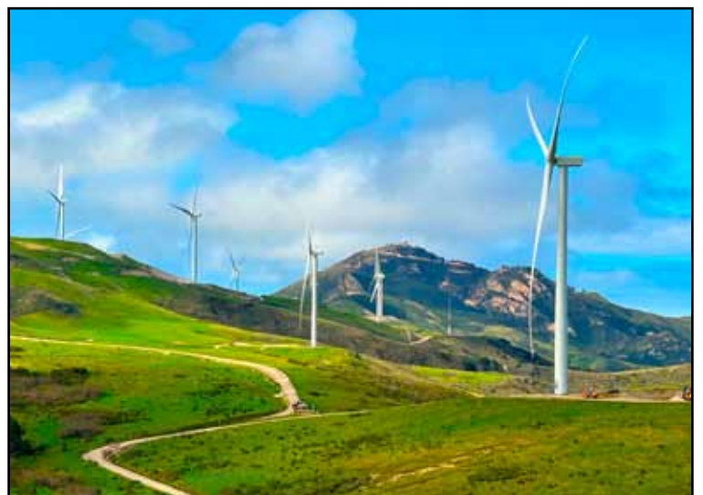
No more oil indeed. Instead, let's seriously consider a strong effort for renewables, such as these wind turbines. Sierra Club and community leaders attended the Strauss Wind Project ribbon cutting on Feb. 29 outside Lompoc. It has 27 turbines, powers 400,000 homes day and night. (Photo by Jon Ullman)
