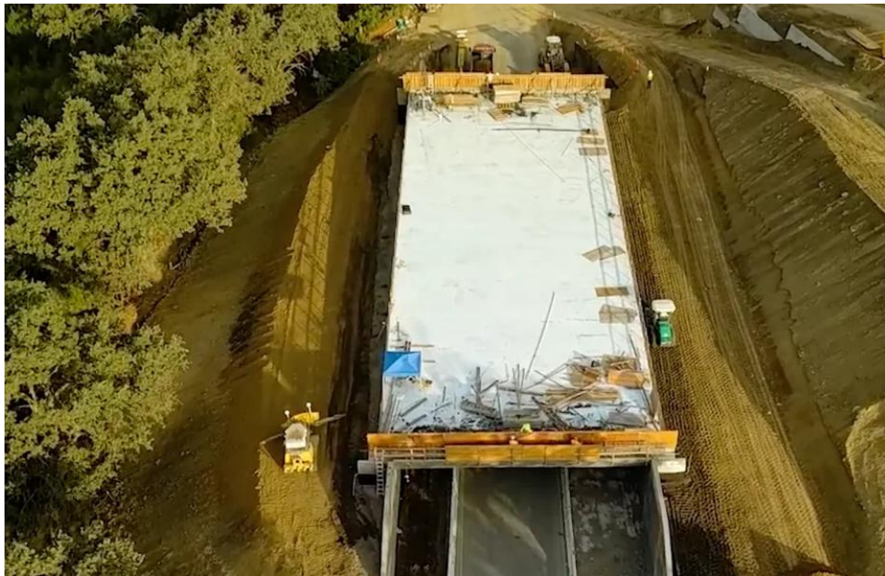
Wallis Annenberg Wildlife Crossing undergoing construction
