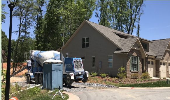
Tons of concrete were delivered daily.
