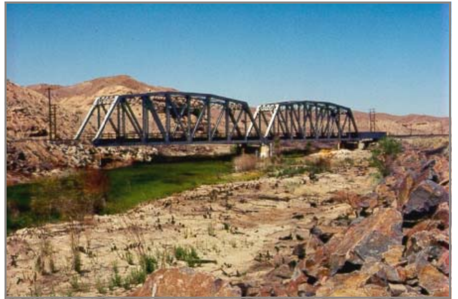
Mojave River in Afton Canyon Natural Area
