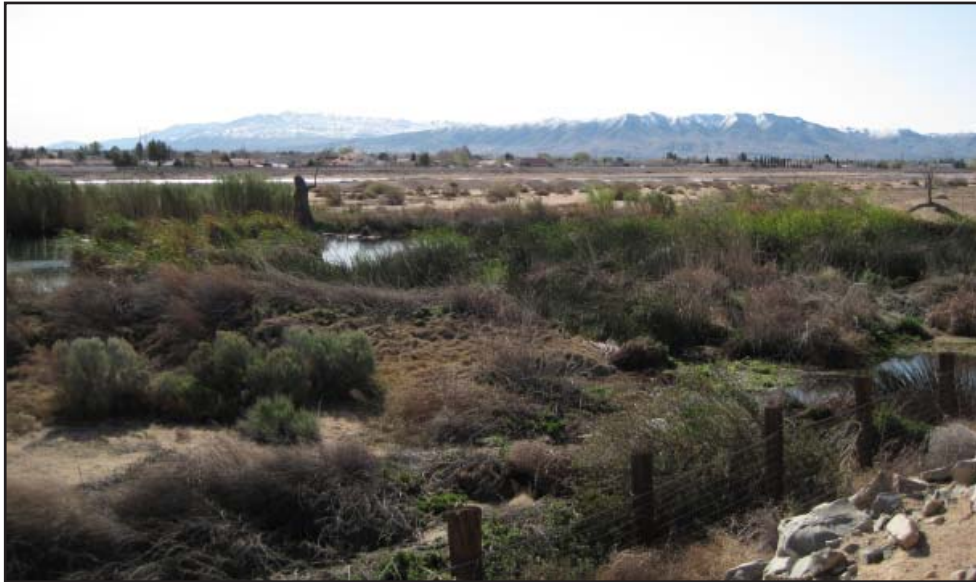
220Kv power lines crossing Roundup Way in Apple Valley.
