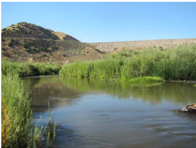
This quiet pool in the Mojave River is the result of a beaver dam below the "spillway." Saddledye embankment (Mojave River dam) is in the background. Photo by Jenny Wilder
