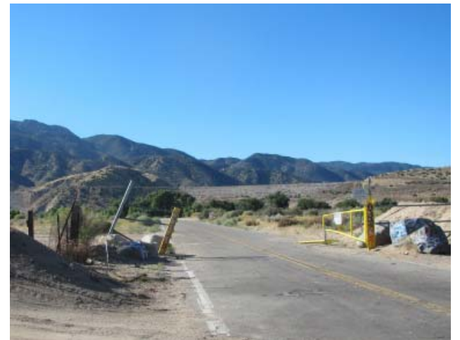
This gate, at the end of Deep Creek Road, was re-installed in the spring and has now been ripped off the hinges again, after the fences at the left were cut. Photo by Jenny Wilder
