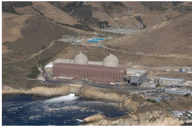
Diablo Canyon Nuclear Power Plant (December 2006)
