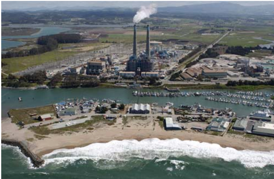
Moss Landing Power Plant/Cal-Am "test" Desalination Facility (December 2006)
