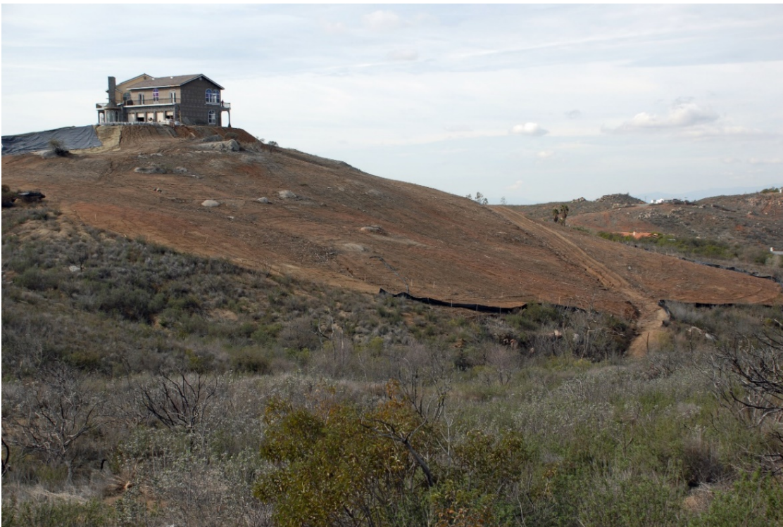
Figure 11. Three-hundred Feet of Clearance. Such bare ground can create a potential “bowling alley” effect, directing embers directly at the structure.
