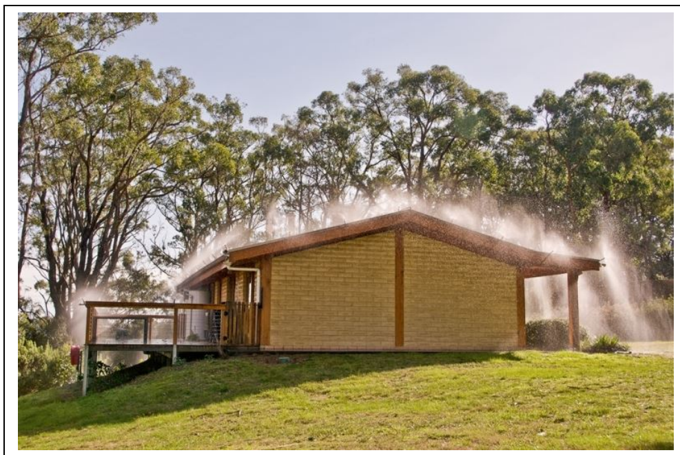
Figure 10. Exterior Sprinklers. As a wildfire approaches, exterior sprinklers wet the structure at risk, the surrounding environment, and increase humidity to prevent ignition. Photo: Platypus Fire Pty Ltd.
