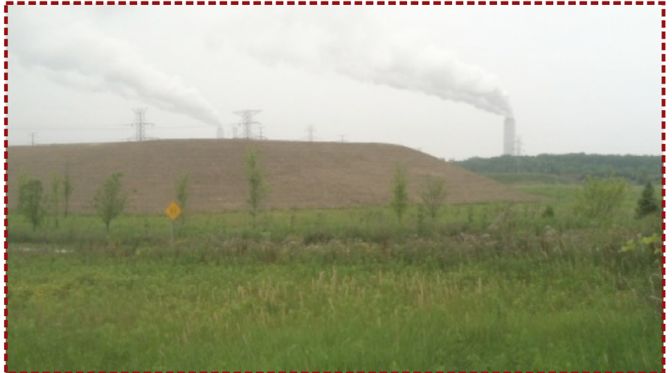
WE Energies Power Plant on Hwy 32
