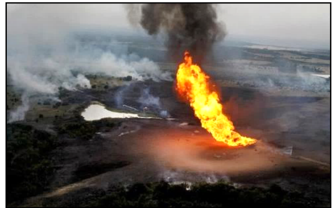
36-inch natural gas pipeline fire near Cleburne TX, 6/7/2010 (one man killed, flames to 1000 ft high). Photo: AP, Dallas Morning News, Courtney Perry theoaklandpress.com/news/officials-investigate-deadly-texas-gas-explosion/article_f75540b3-78aa-5f61-b3c6-
