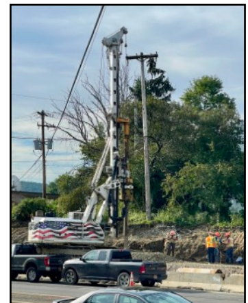
Current construction, Town of Vestal portion
