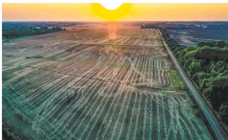
Preparing the way for Blue Oval City. Photo courtesy of Patrick Lantrip/ The Daily Memphian .
