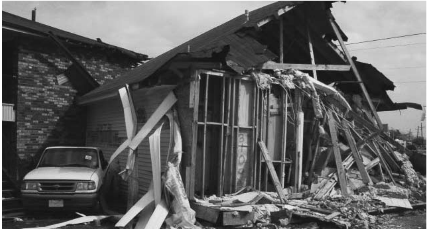
New Orleans devastation wrought by Hurricane Katrina.
