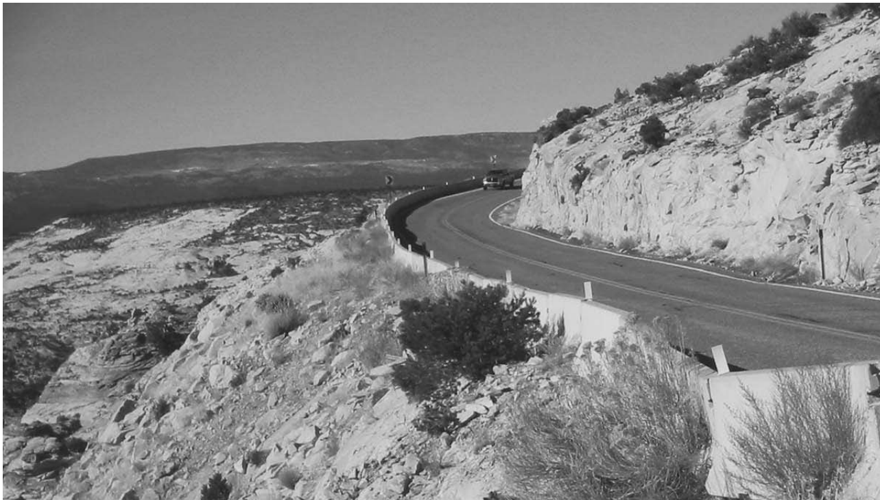
Failing Jersey barriers.
