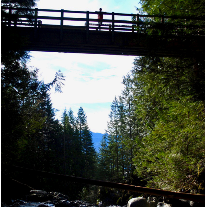
Footbridge above Wallace Falls
