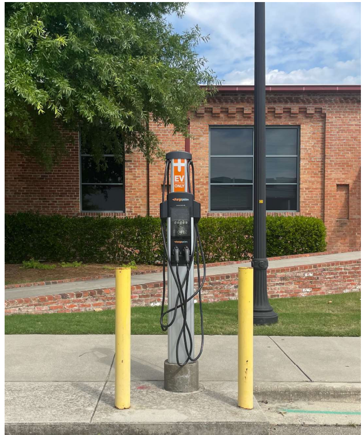
Image: Level 2 EV charging station off of Blackwell street in Durham; Shanya Hayes.
