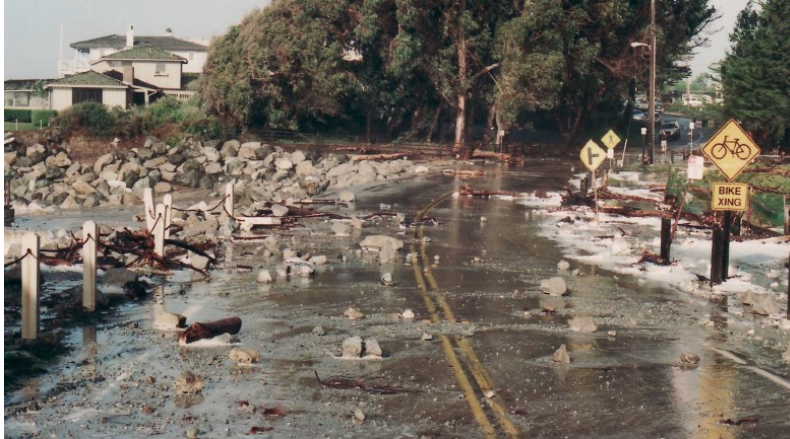
Rocks and debris across East Cliff Drive at the Moran lagoon frontage
