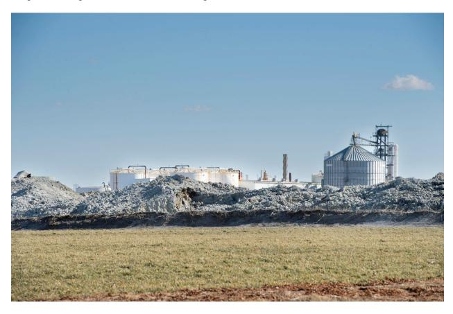
In mid-February, Posi-Shell, a combination of cement, clay and polyester fibers, was applied to a pile of wet cake and sludge produced by the AltEn ethanol plant near Mead. Journal Star file photo
