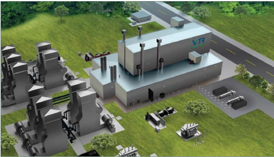
A rendering of the Versatile Test Reactor proposed in Idaho. It would be the first sodium-cooled fast test reactor built in the U.S. PHOTO COURTESY OF THE U.S. DEPARTMENT OF ENERGY.
