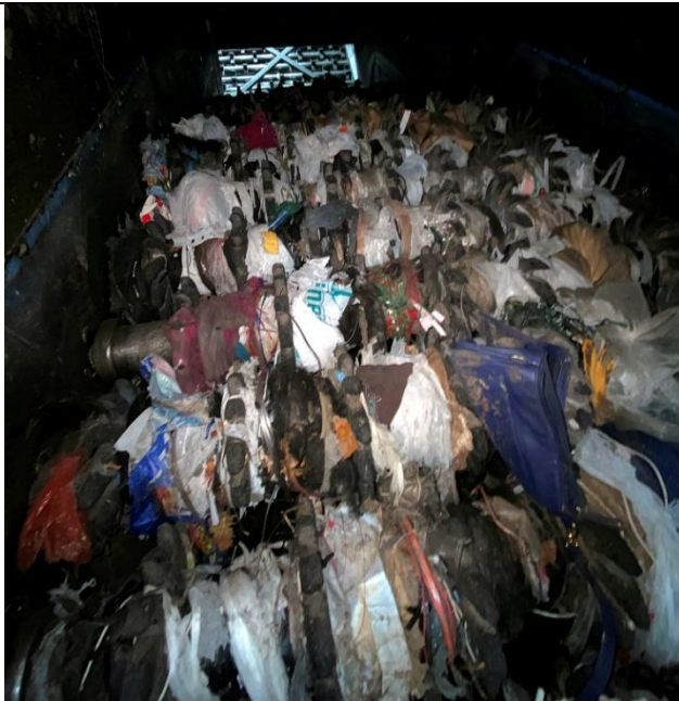
Fouled screens at the end of the day
