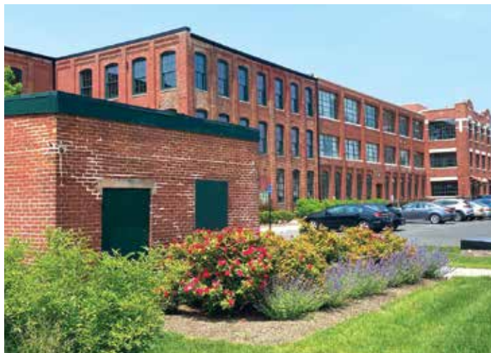
The NJ Chapter offices are now in a repurposed former luggage and clothing factory.
