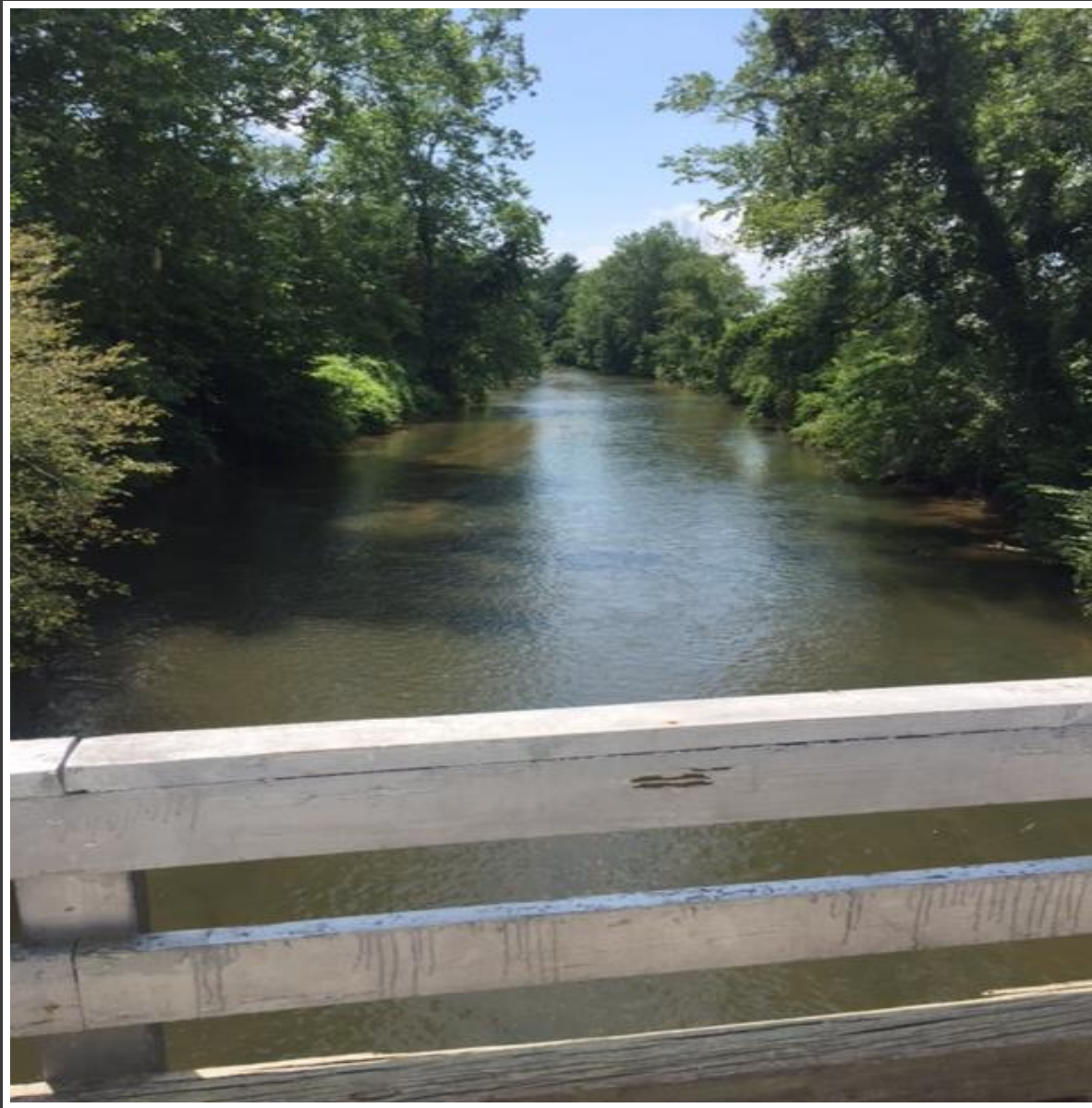
Green Rd. Bridge Looking Upstream
