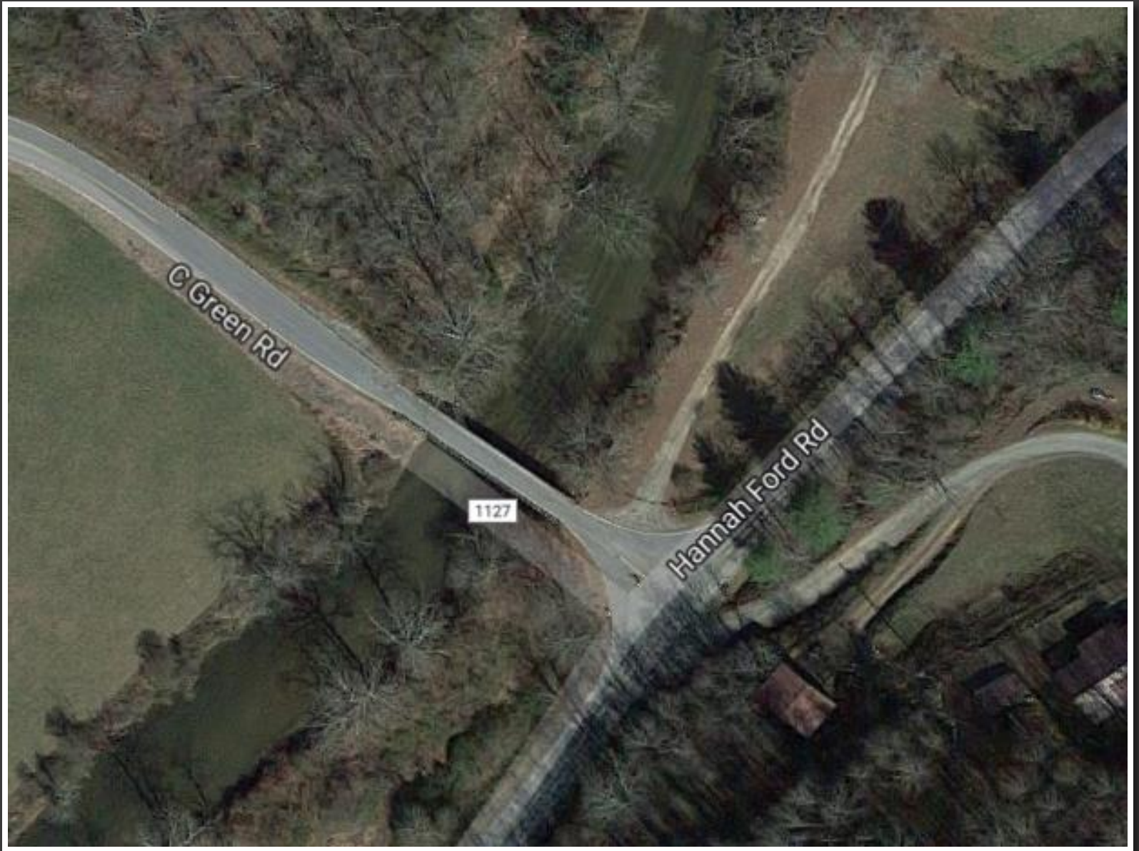
Green Rd. Bridge
