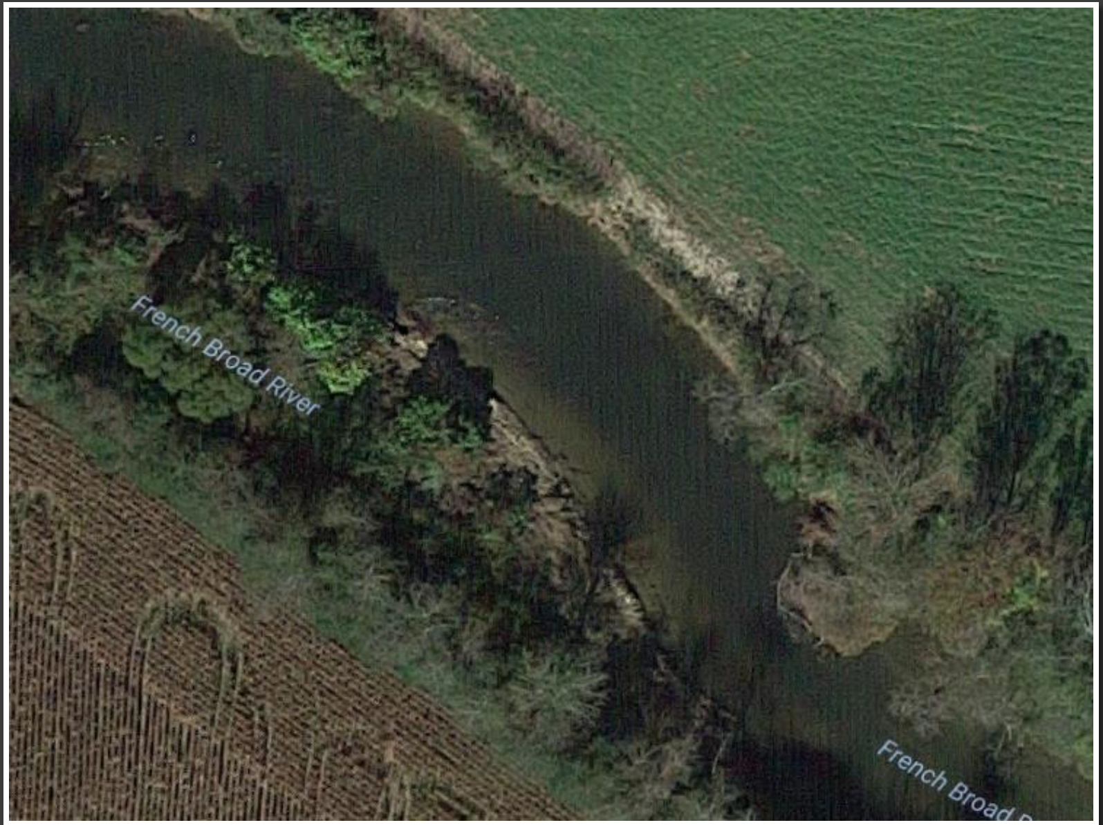
Deep Channel in Center of River: Channelization effects, even 130 years after construction.
