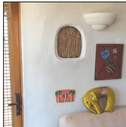
A window in the wall provides a glimpse of the home's hay-bale insulation.
