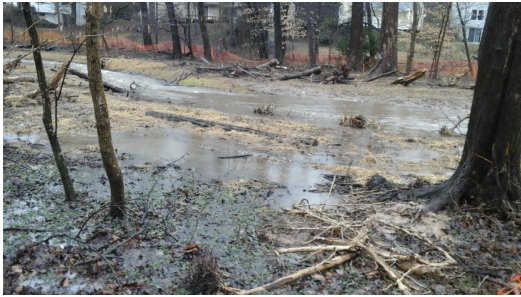
Newly Restored Stream Connecting to the Engineered Floodplain
