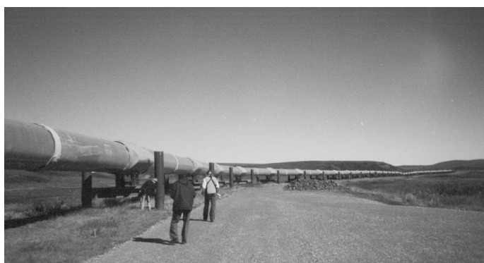
The pipeline: one short section between the Brooks Range and Fairbanks. All of the pipe's 800 miles were made in Japan.
