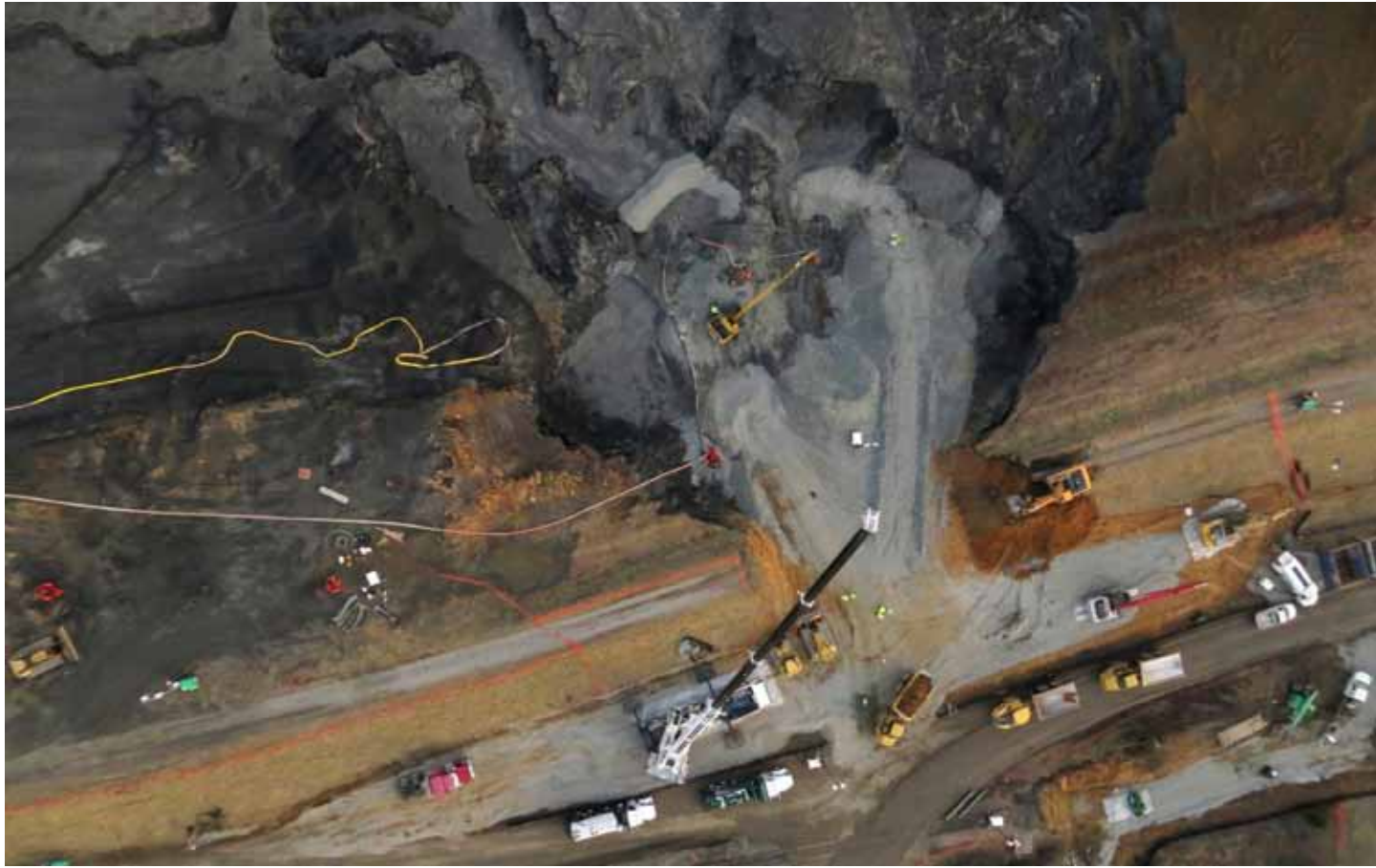
IN MARCH OF 2014, A DUKE ENERGY COAL ASH IMPOUNDMENT FAILED AND SPILLED MORE THAN 39,000 TONS OF COAL ASH INTO NORTH CAROLINA'S DAN RIVER
