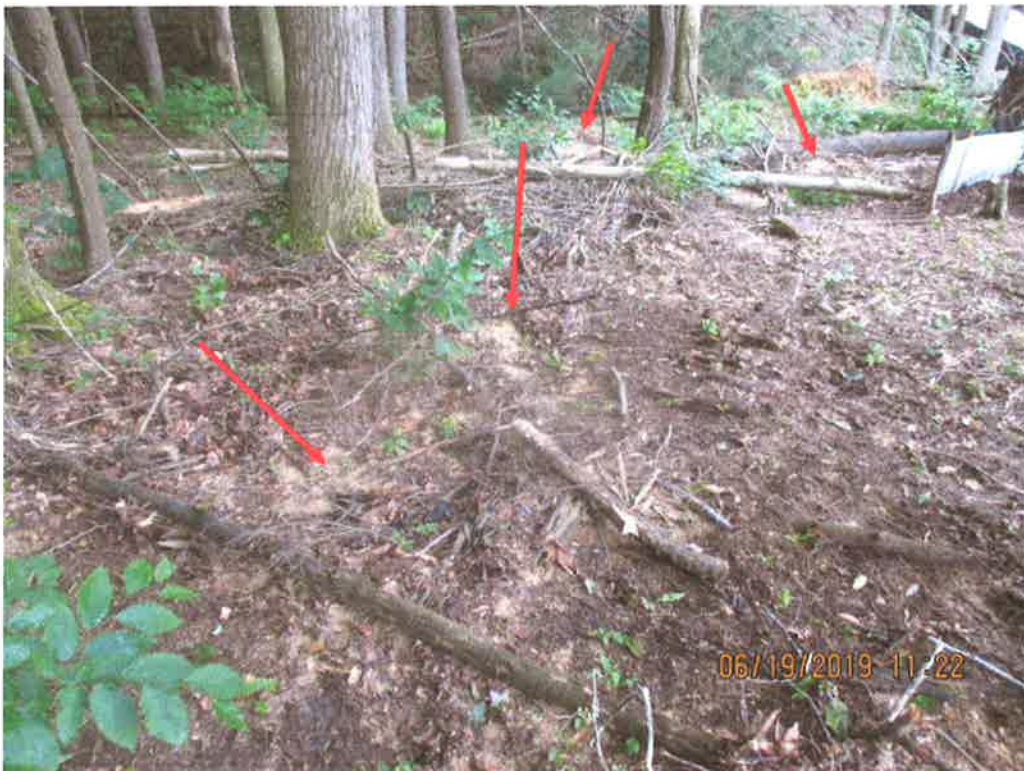
Downslope of Waterbar outlet controls at Station No. 6587+00. Arrow depicts Sediment Deposits.
