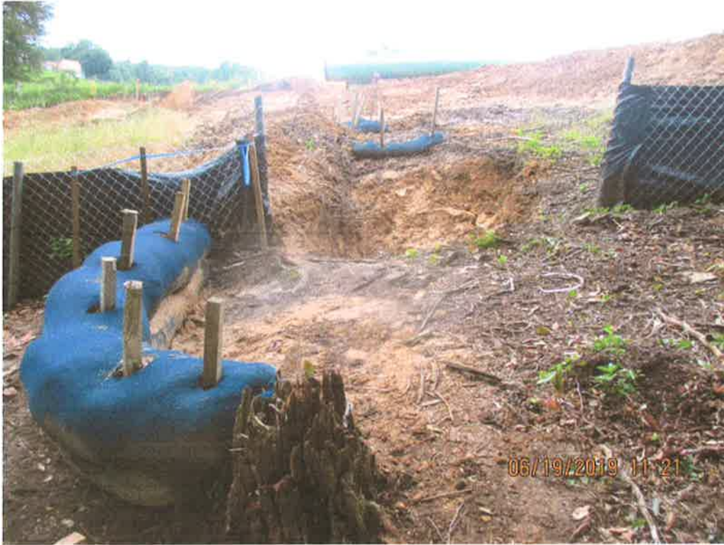
Waterbar Outlet and primary controls at Station No. 6587+00 facing towards Additional Workspace and CR 18.
